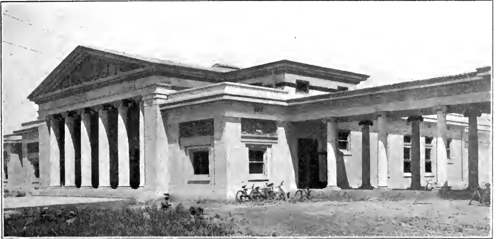
The New Anaheim Union High School.
